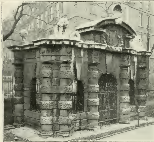
THE WATER GATE OF YORK HOUSE.
